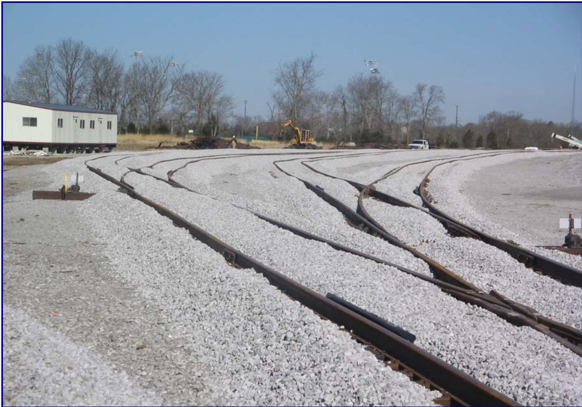
March 15, 2006 – Track Construction for the Lebanon Layover Facility
