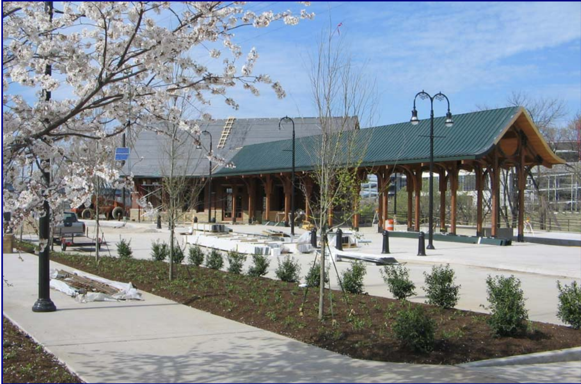
March 27, 2006 – Masonry Work at Riverfront Station
